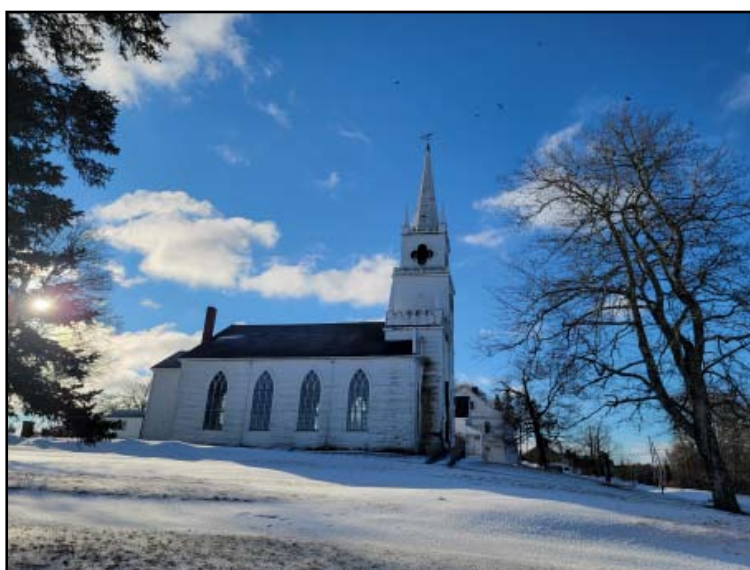
The First Congregational Church of East Machias is one of the only examples of Carpenter Gothic architecture in Maine. A group of devoted volunteers is raising money to save the structure, which is considered one of the "most threatened architectural resources in the state of Maine." Submitted photo
