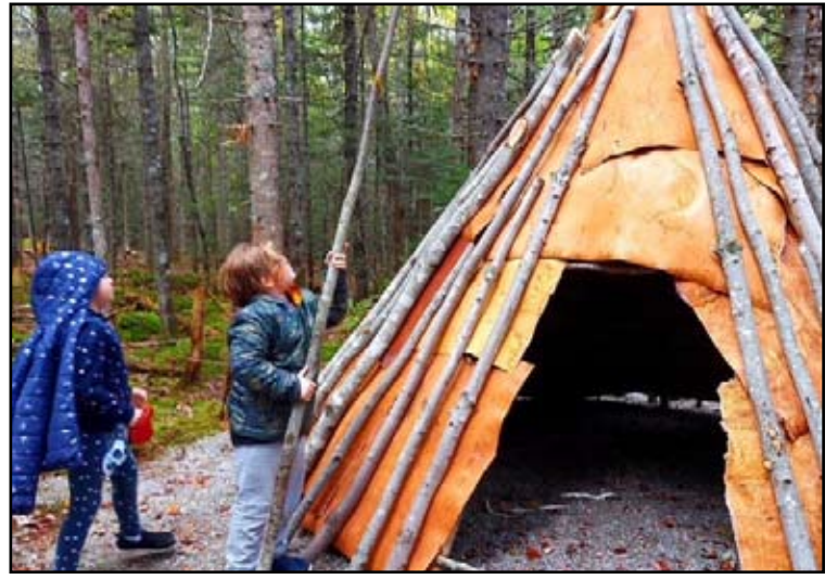
Honoring tribal culture, history, and artistry is important to the Langleys, who attempted to build a representation of a Wabanaki wigwam using their own birch bark, which turned out to be brittle due to its proximity to salt water. New birch bark has been ordered, and they hope to begin construction again soon. Submitted photo
