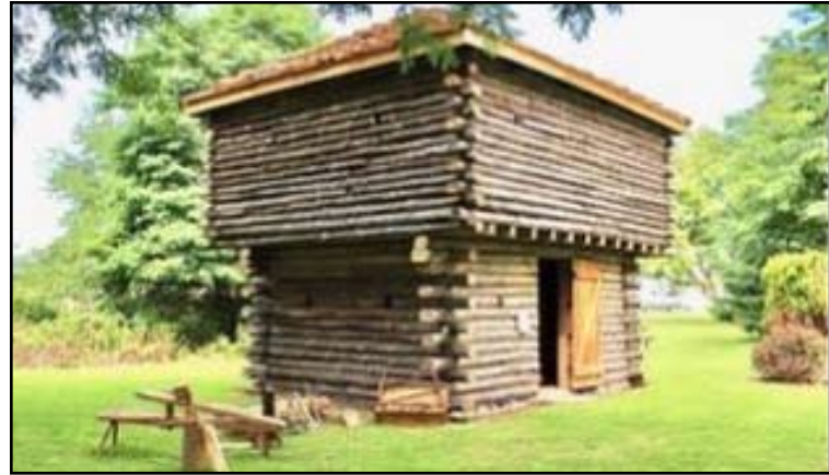
Linda and Arthur Langley plan to begin construction soon on a historic blockhouse fort, like this one, to enhance their property as a site for historical reenactor gatherings. Submitted photo
